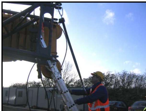
Figure 3 - Fall Arrest System
