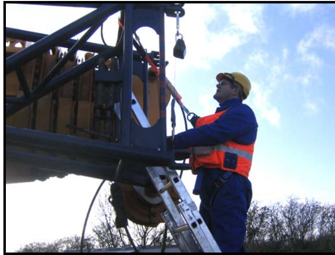
Figure 2 - Work Positioning System
